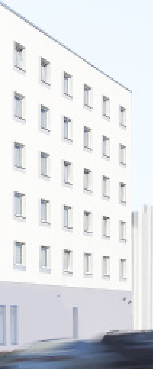
First Hotel complete constructed in modular design in Russia. Six floors with 145 double rooms.
